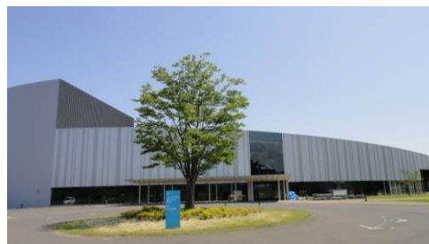
Yugakukan Emergency Shelter Unusually for an emergency shelter, it has both heating and air conditioning.
